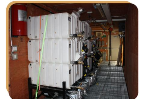
This is a 30 ft container mobile lube room designed based on lubricant usage of a client in the mining industry. It contains 8 Des-Case LT-LMS oil storage systems (Des-Case LT-Series Lubricant Management System), with fire suppression, insulation, heating, ventilation, electrical, chain hoist, and roll-up door.
